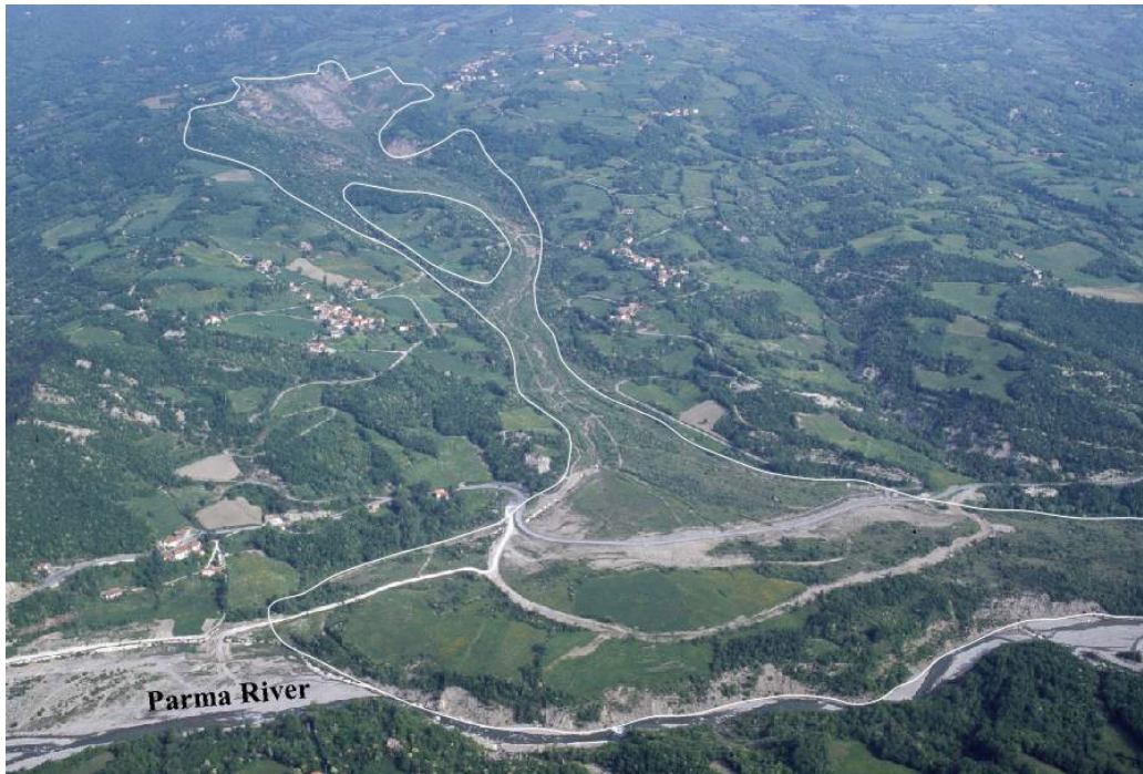
Figure 2. The ancient Signatico earth flow in Val Parma resumed activity in 879, 1710, 1836, 1879, 1896, 1901, 1905, 1906, 1945, 1947, 1948, 1949, 1957 1977 and 1999. In consequence of 1836, 1879, 1896 and 1945 events, it obstructed the valley floor and large lakes formed. Photo by Bertolini G., 2006.
