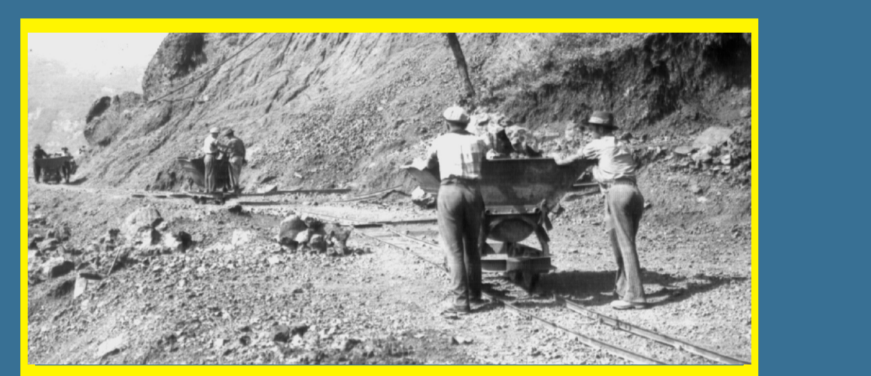
An historical view of the quarrying work
