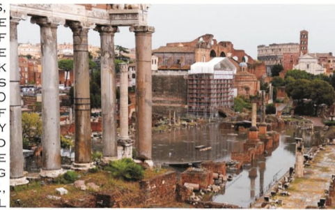
FIGURE 1: FLOODING OF ROMAN FORUM DURING 20 OCTOBER 2011
