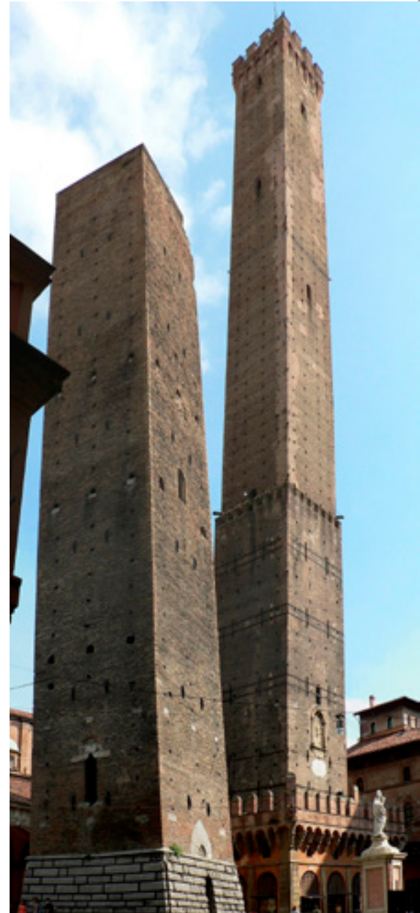
Fig. 1 Selenite is the basement of Towers of Asinelli (97,2 m ) and Garisenda Towers (47 m) (XII century). They are the symbol of the city of Bologna and are both leaning 2.23 m and 3.22 m respectively. The names are derived from families that built them.
