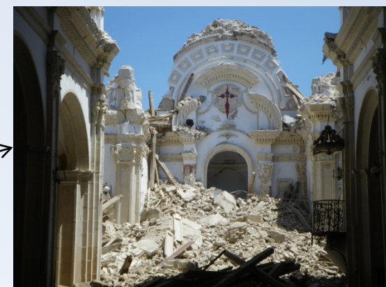
Photos from Lorca earthquake
