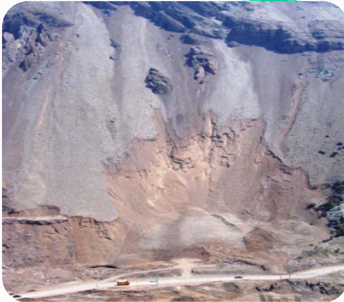
A general view of third station (Haji Abad)
