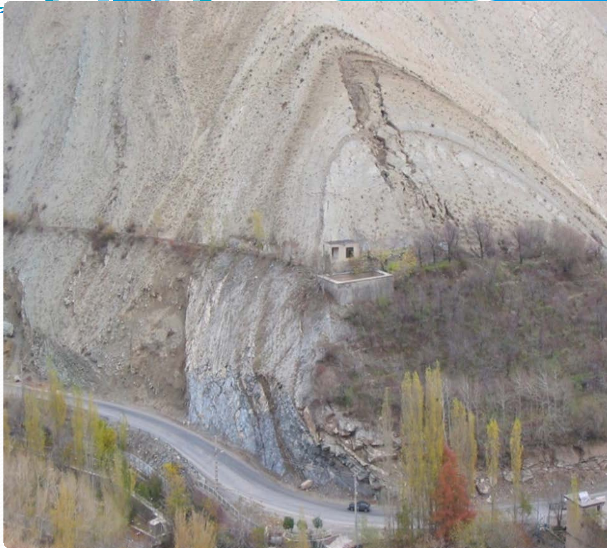
A general view of station 4 (Maygon area).
