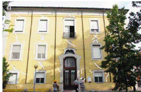
Fig. 8. Examples of “uniform” global mechanism (with the localization of damage in spandrels) observed in some buildings in Mirandola (a) and Finale Emilia (b, c): on the left, the main cracks are marked in white on a general view of walls; on the right, some particular of cracks on spandrels are shown.
