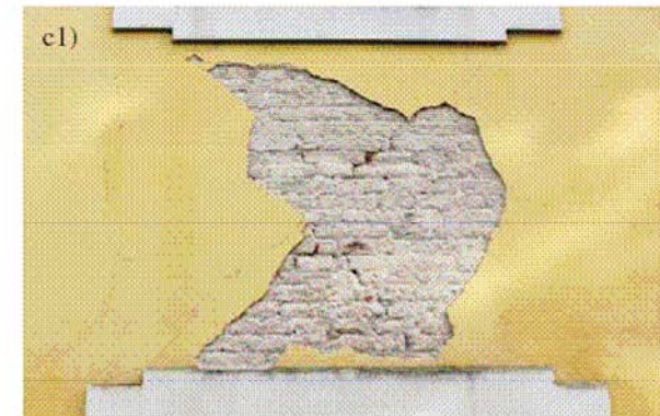
Fig. 8. Examples of “uniform” global mechanism (with the localization of damage in spandrels) observed in some buildings in Mirandola (a) and Finale Emilia (b, c): on the left, the main cracks are marked in white on a general view of walls; on the right, some particular of cracks on spandrels are shown.
