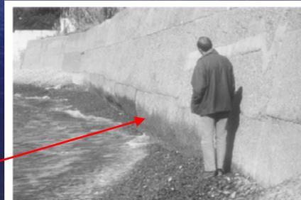
Fig. 15. Eighteen year old concrete sea wall at Torre Calce with a 50 cm head notch.
