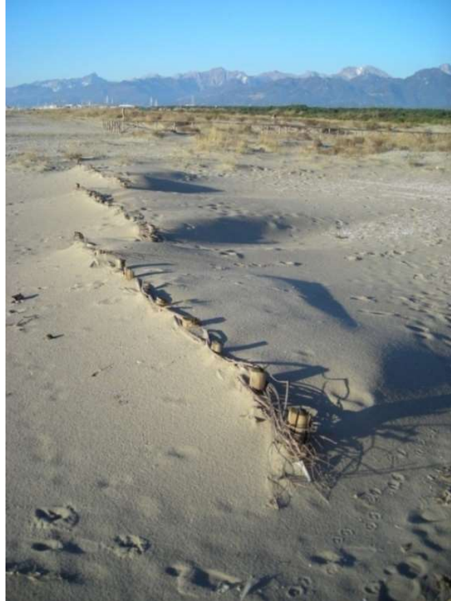
Viminate built in Marina di Vecchiano (Pisa), for the closure of bow-outs in the dune system. (year 2009).
