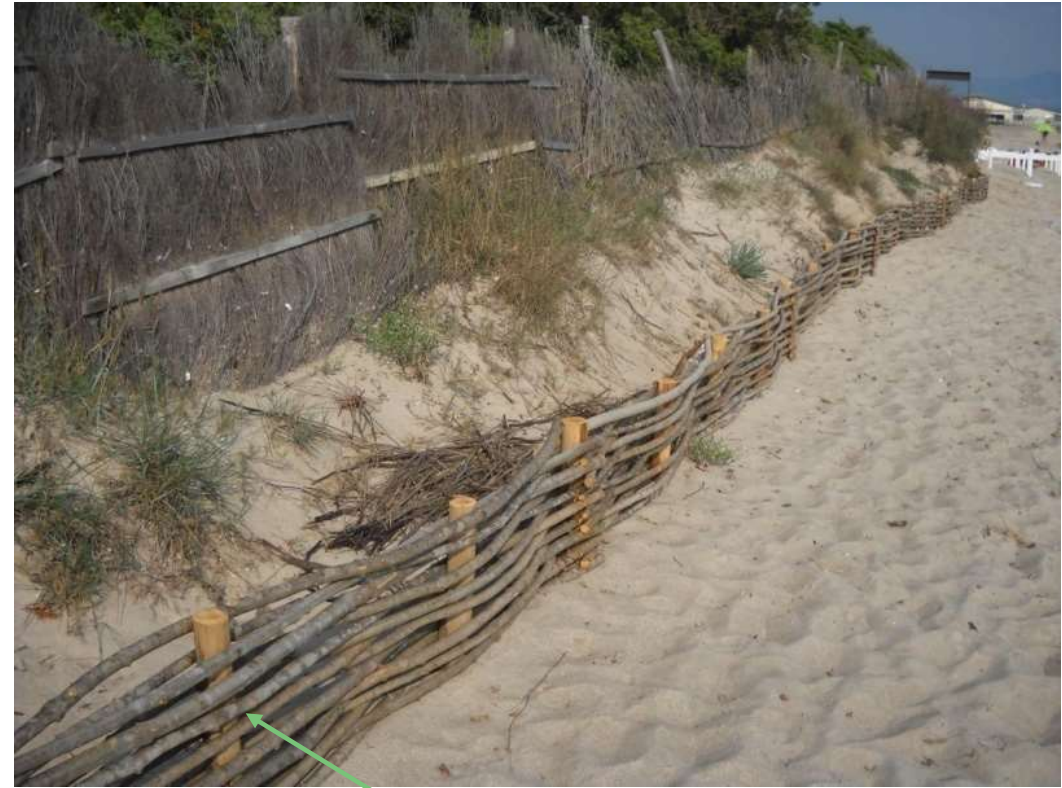
Viminate built at the foot of the dune in Carlappiano (Sterpaia)
