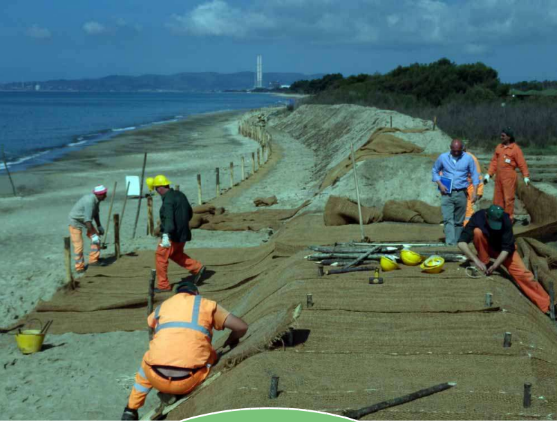
Dune Reconstruction with Reinforced Sand
