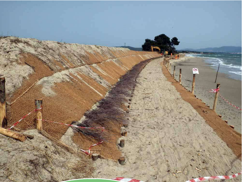
Coconut Fiber Network Tamarix L. Cutting
