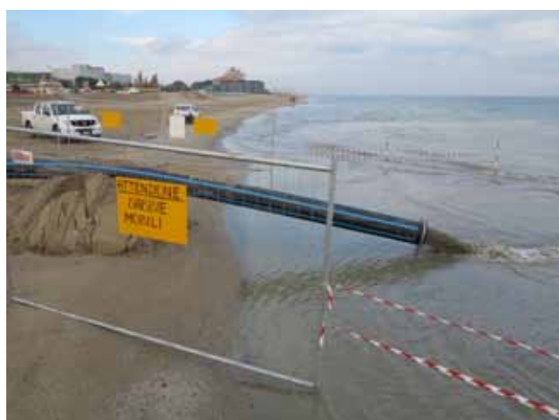
Figure 31 Nourishment with the sand-water mixture coming from the Riccione port dredging.
