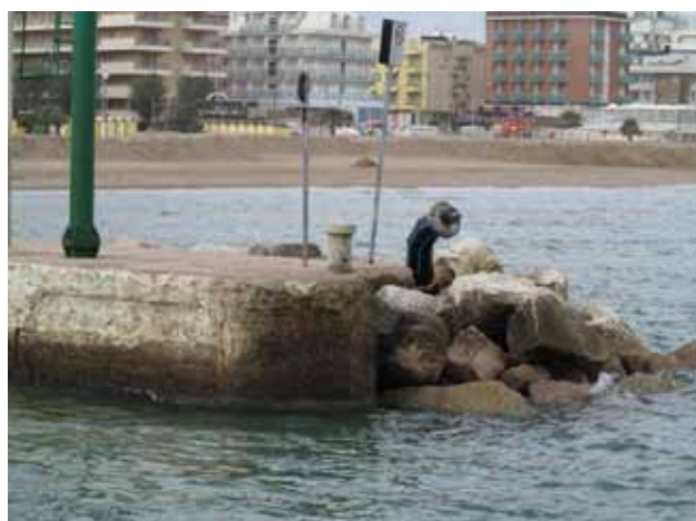
Figure 30 Joint plug of the Riccione sand pipeline
