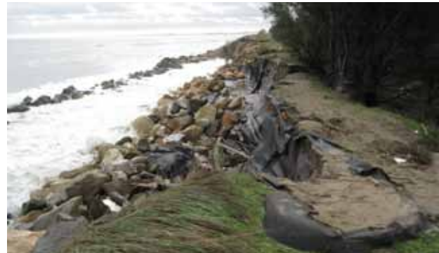
Figure 15 Seawall eroded near the Volano nord pinewood.
