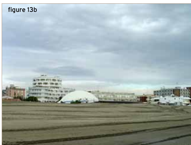
figure 13 A: not properly built winter defence embankments, by removing sand from the foreshore. B: properly built winter defence embankments, with sand coming from other sources
