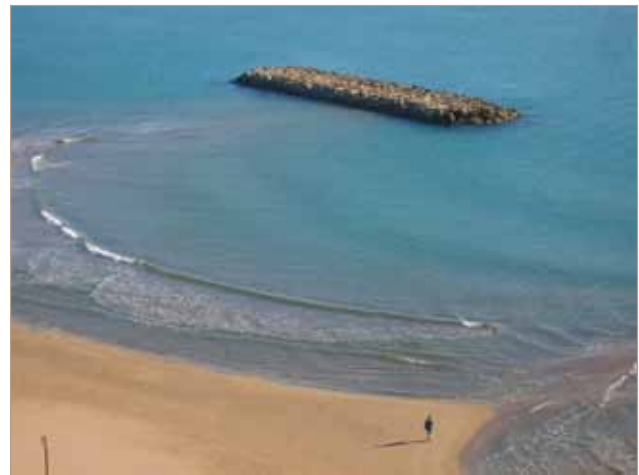
figure 22 Tombolo behind breakwaters
