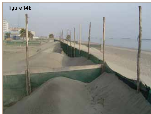
figure 14 A: negative effects caused by the absence of windbreaks B: a windbreaks properly built
