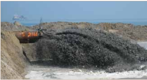
figura 24 Pipeline working during the second off-shore sand nourishment in 2002.
