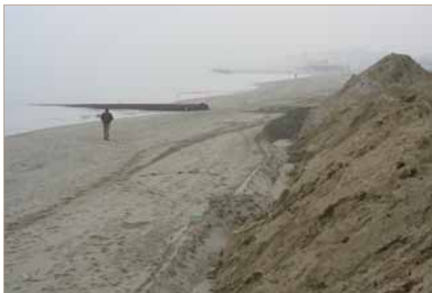
figure 26 South of Riccione: sand coming from the building excavation before nourishment by means of off-shore sand in spring 2007
